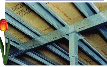
ALL IN 65mm x 65mm x 2mm HOT DIPPED GALVANISED STEEL WITH BOLT DOWN FOOT WHICH CAN BE CAST IN CONCRETE
